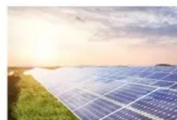
Energy Storage System
