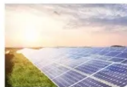
Energy Storage System
